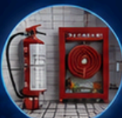
FIRE SAFETY SYSTEMS
